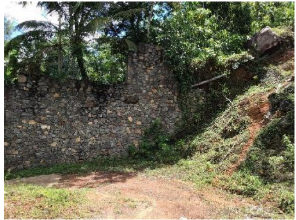
Retaining wall constructed near mitigation area
